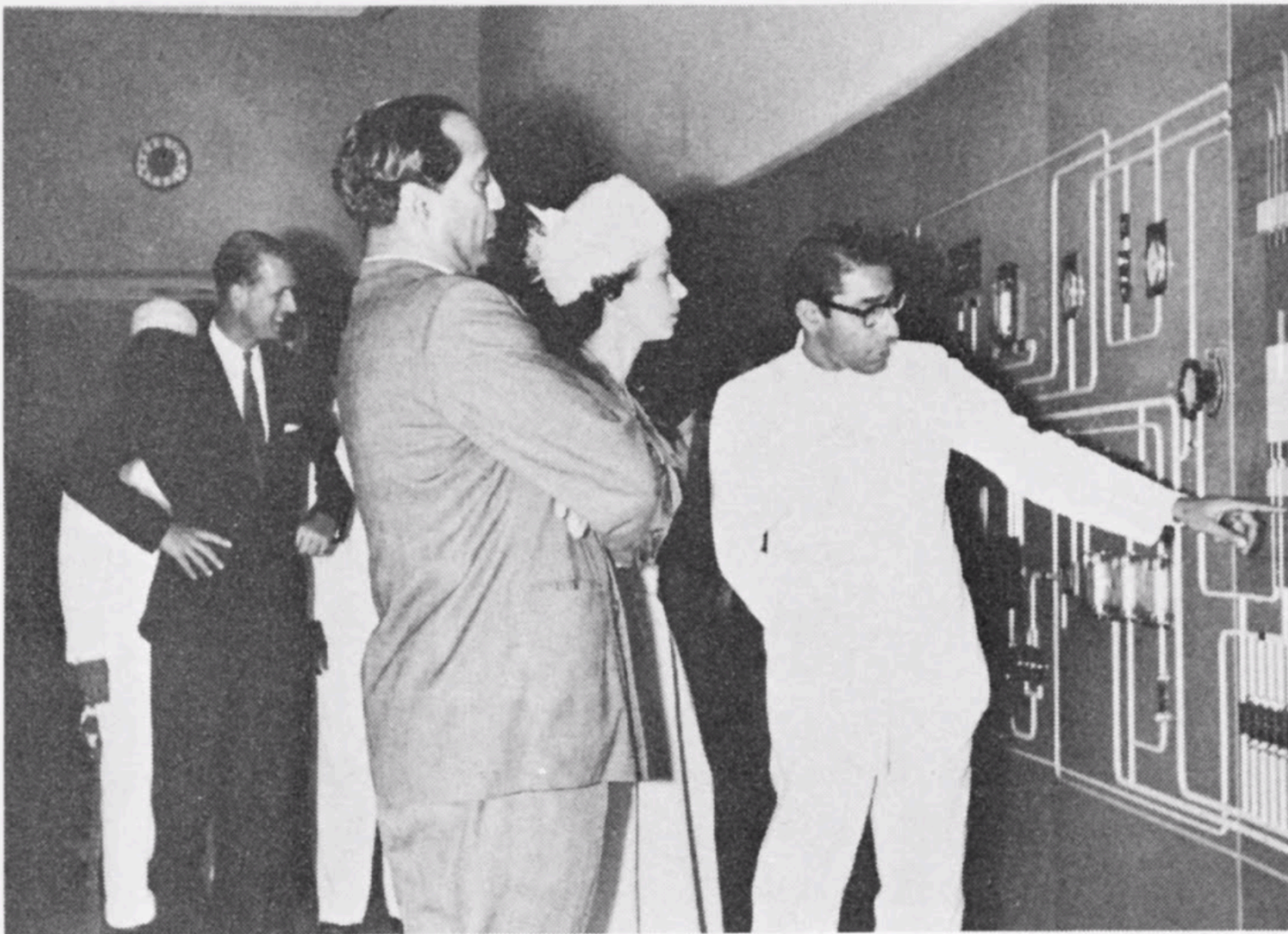
Her Majesty Queen Elizabeth is shown the control panel at the Canada-India Reactor, built at Trombay, India, as a joint project of Canada and India under the Colombo Plan.
